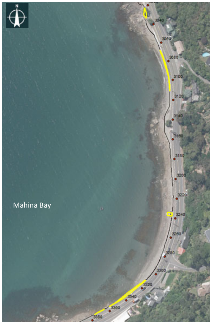
Figure 5-1: Example de-reclaimed area within Mahina Bay. Yellow outline shows area between existing seawall toe and new seawall toe to be returned to the coastal zone. Numbered annotations indicate Project chainage. [Source: Eos Ecology 2018 and project data].
