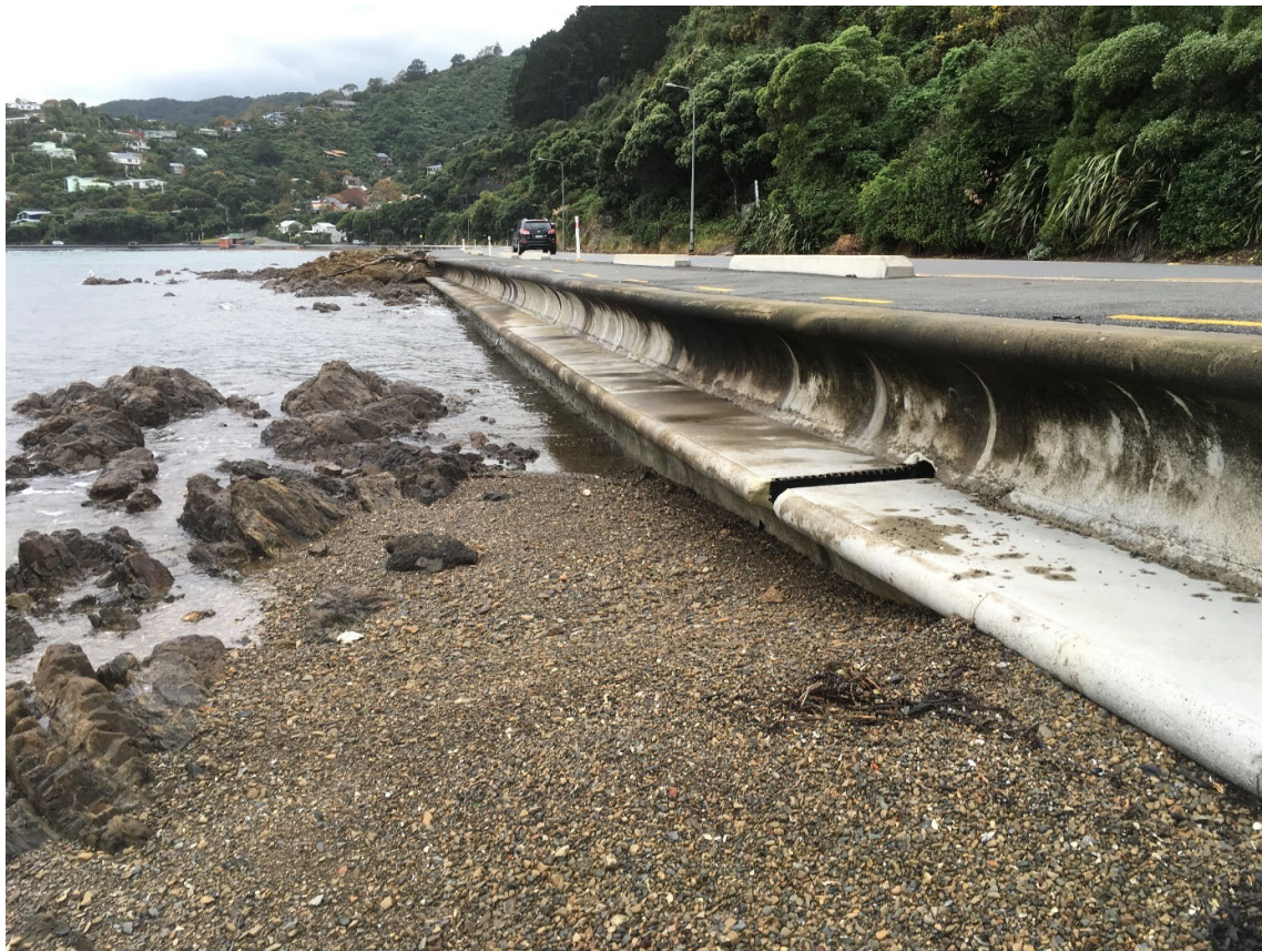
Figure 4-6: Modern double curved seawall at southern York Bay. [Credit: 25/12/2017, M. Allis (NIWA)].
