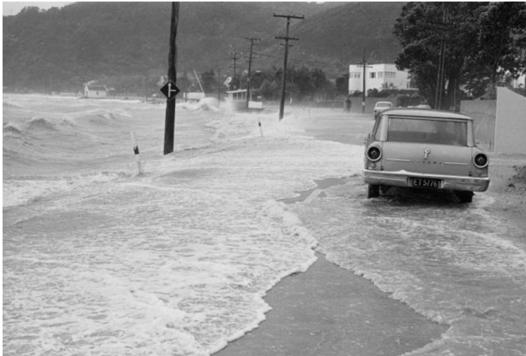
Figure 4-22: Wave overtopping at southern Lowry Bay (8 May 1969). [Source: 18 ].
