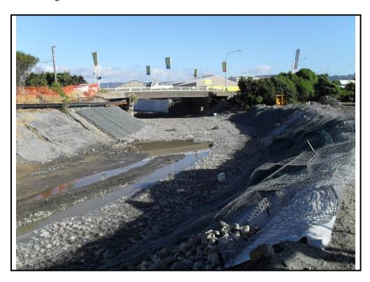
Photograph 4: Cell H looking downstream towards Seaview Road Bridge, following the removal of contaminated material and during the installation of reno matresses.
