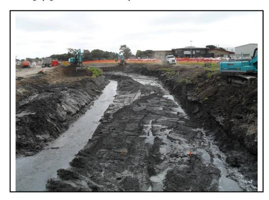
Photograph 4: Cell A looking downstream post-excavation. Orange pegs denote validation sample locations.
