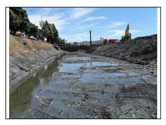
Photograph 5: Looking downstream towards coffer dam 5 following excavation.
