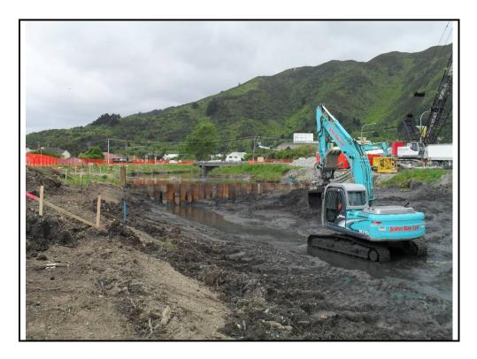
Photograph 2: Looking upstream towards Coffer Dam 1 during excavation.
