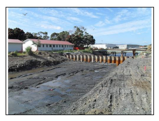
Photograph 3: Looking upstream towards coffer dam 2 following excavation.
