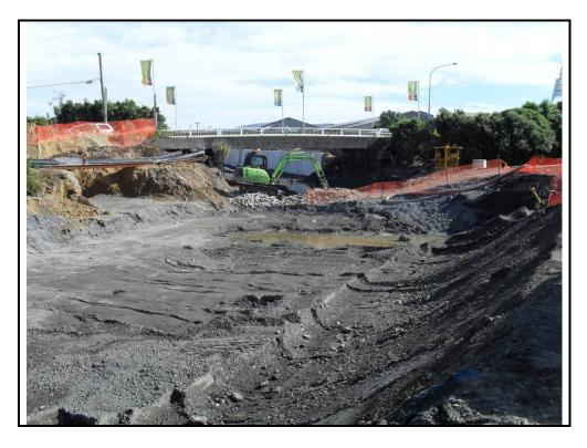
Photograph 3: Cell H looking downstream towards Seaview Road Bridge, following the removal of contaminated material.
