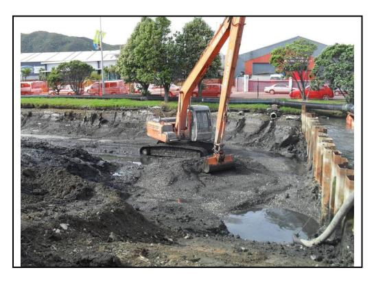
Photograph 3: Cell E at coffer dam 5 during excavation.
