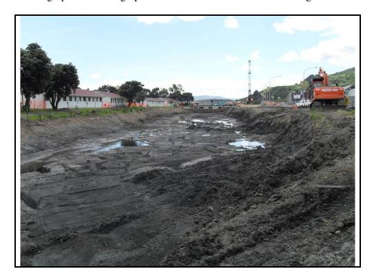
Photograph 4: Looking upstream towards coffer dam 2 following excavation.
