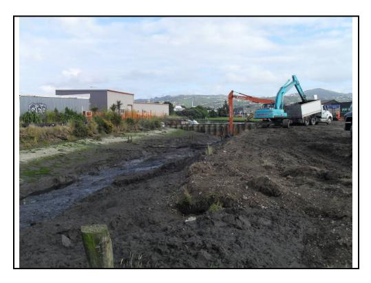
Photograph 1: View looking downstream towards coffer dam 7 during the removal of contaminated material.
