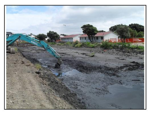
Photograph 1: Cell C during the early stages of excavation. Coffer dam 3 (in background) was removed during the works.
