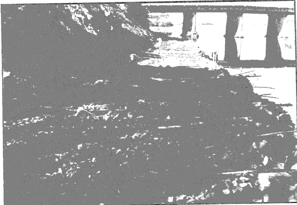
Plate 103: Reinstatement of the eastern bank, Ewen Bridge 1985.
