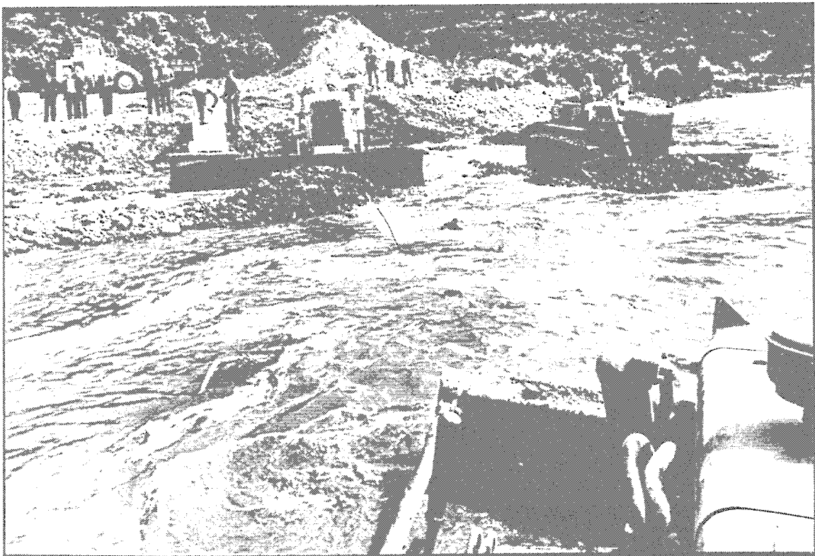
Plate 93: Closing the channel to direct water through the first stage, Nov 1969.
