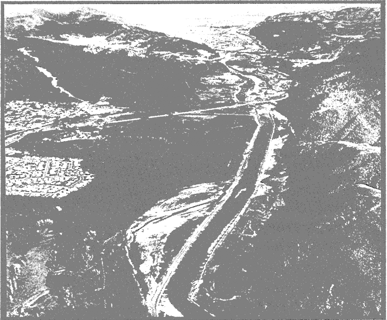
Plate 94: Aerial view of the combined first and second stages of the Silverstream Cut.
