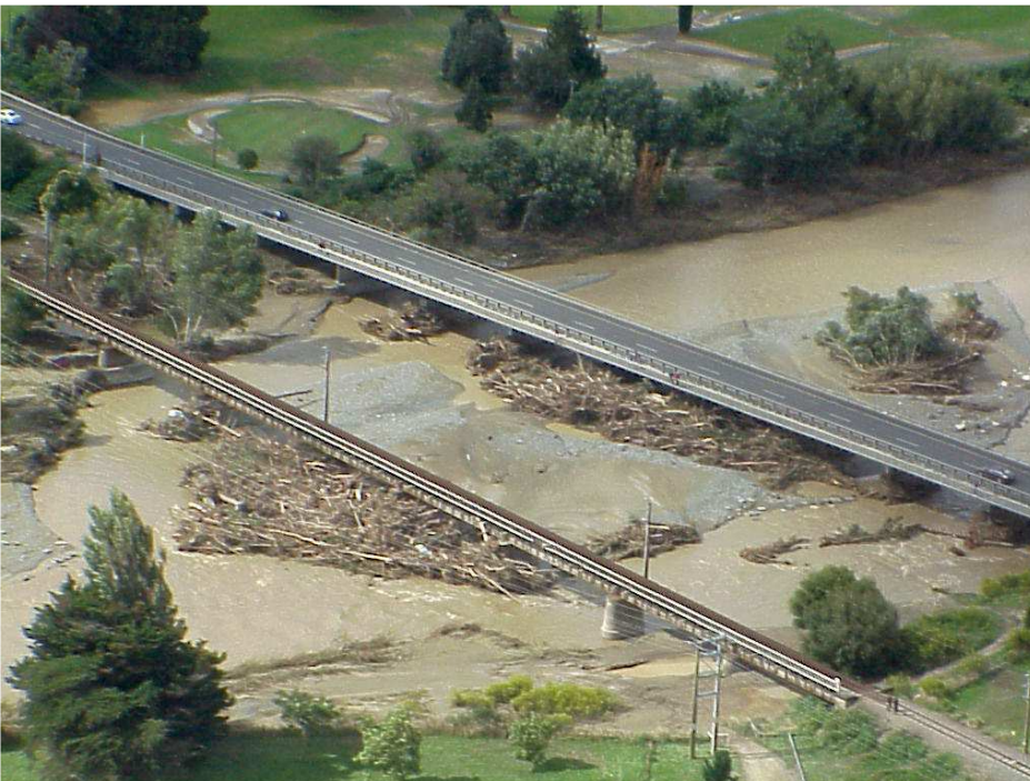
Photo 2 - SH54 Aorangi road and rail bridges over the Oroua River, Fielding, February 2004. Permission of Civil Defence
