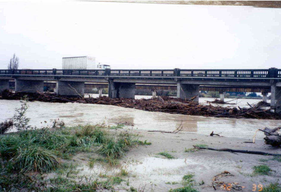
Photo 1 - Wairau river, Marlborough over SH1 (May 1995). Falling stage of about a 2-year return period flood (photograph courtesy of Brin Williman).
